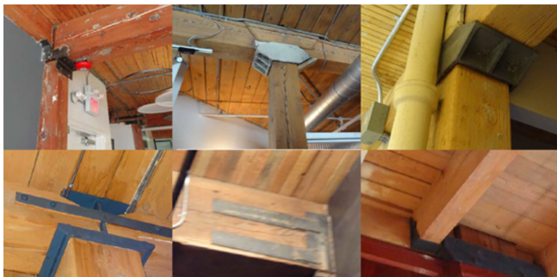
Figure 2.2. Typical historic post and beam connections (from Appendix C-2, Koo, 2013). Metal castings provide end-grain bearing to reduce the effects of wood shrinkage.
