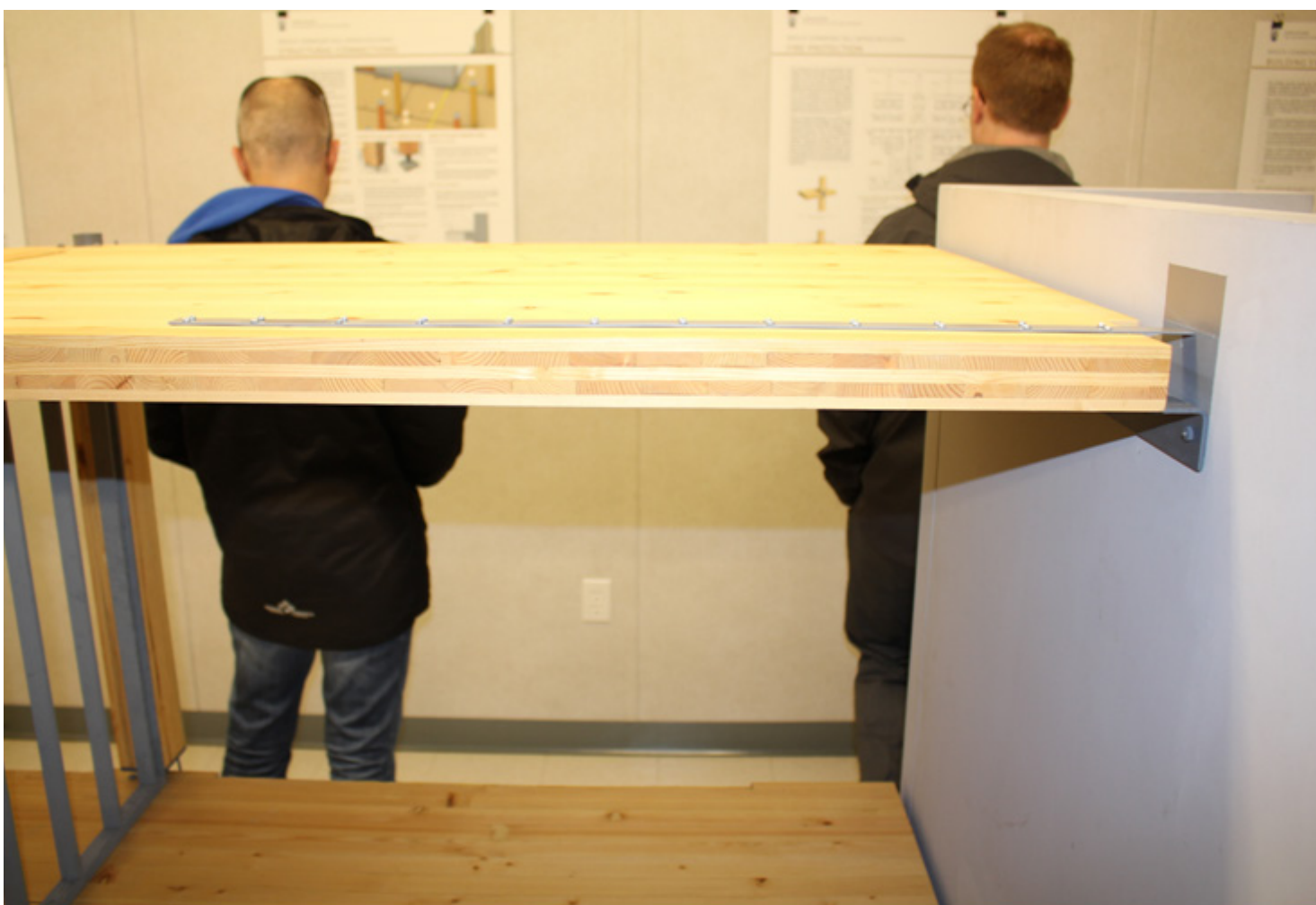
Figure 4.7. UBC Brock Commons demonstration connection of a CLT panel to concrete shear wall with tension strap and vertically slotted connection (Photo: D. Moses)
